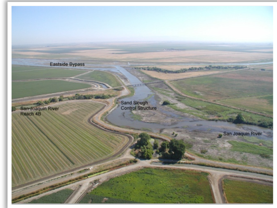
Sand Slough Control Structure
