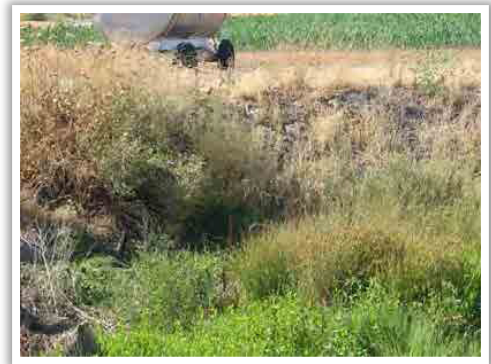
Dense Vegetation at Owen's Creek Diversion, 2012
