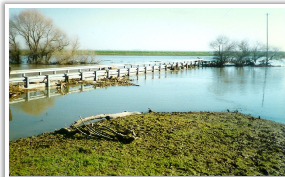
Eastside Bypass Flooding at Greenhouse Bridge Road, 1997
