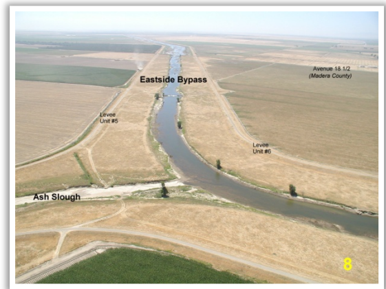
Ash Slough at Eastside Bypass
