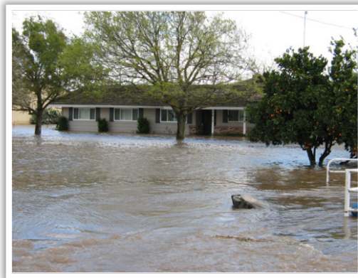
Black Rascal Creek Flooding, 2006
