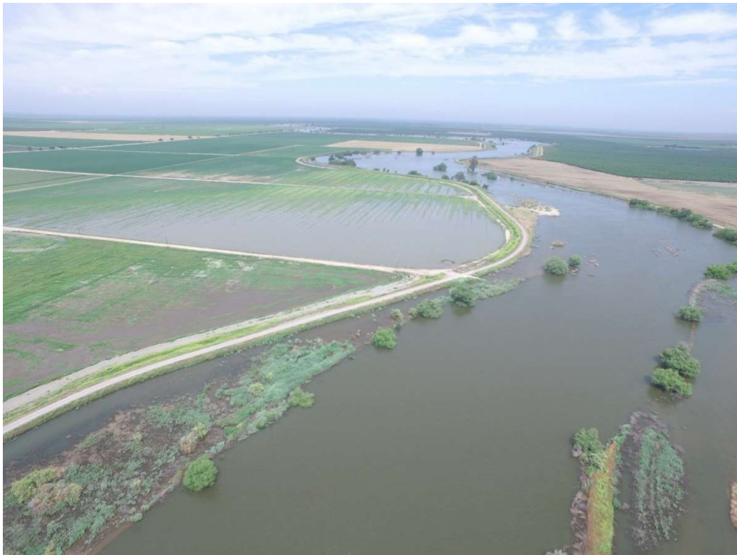
Figure 4-1. High Flows on May 23, 2023 With Seepage Impacts Agricultural Lands North of the San Joaquin River Upstream of the Bifurcation Structure
